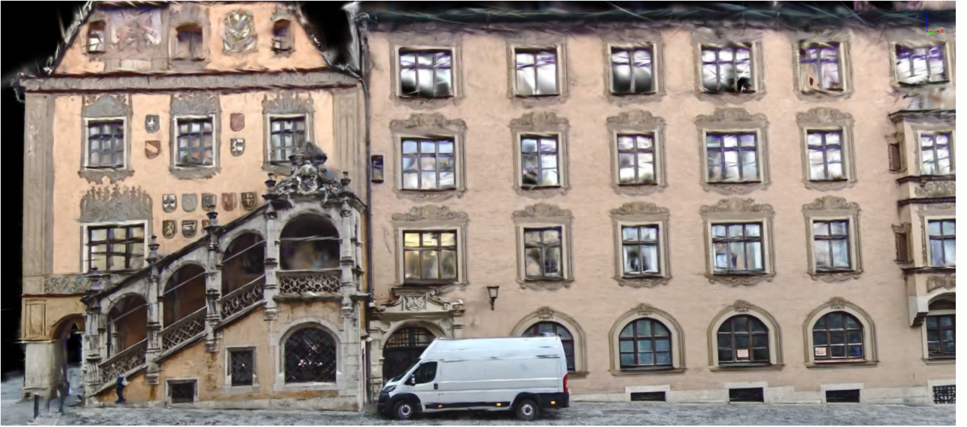
Architectural Facade Scene
